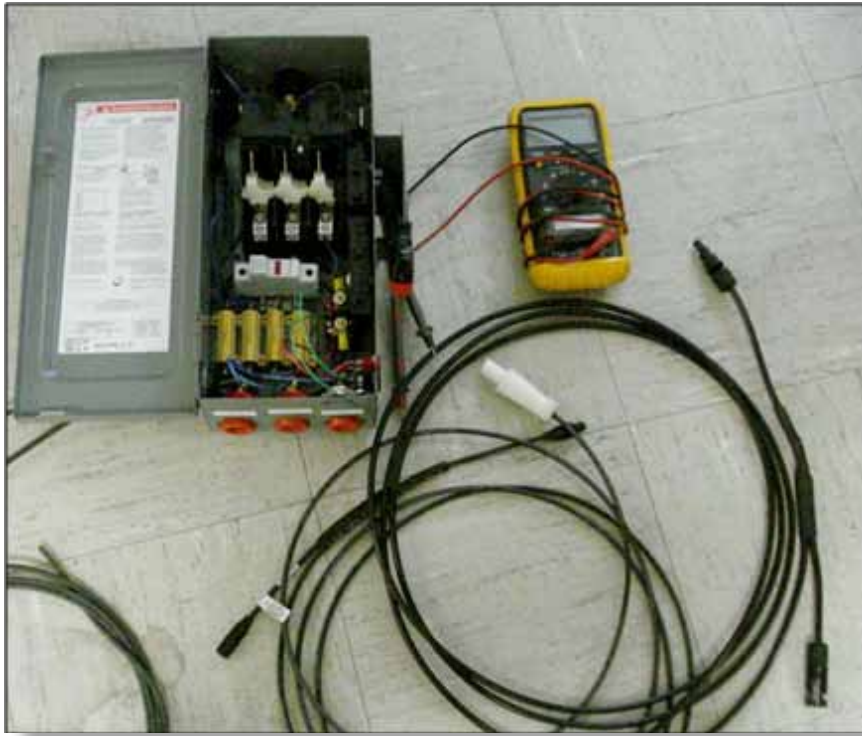
Figure 4. Ground fault appliance with T-cables and meter used to introduce ground faults within an array.
